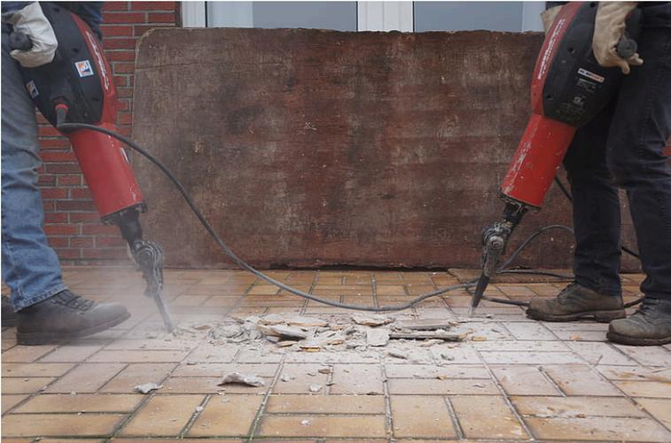
*Figure 9.6: Two workers jackhammering a hard floor*
